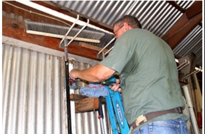
Mark - checking out the wiring
