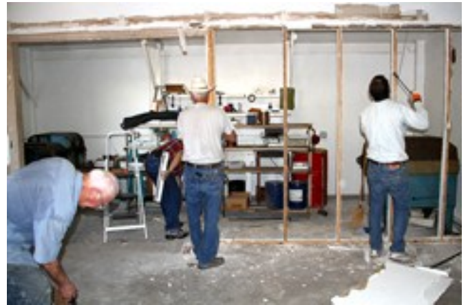
And the wall is nearly gone
