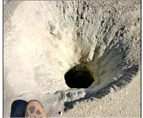
A blasting hole, about 150' deep, add 50' of explosives, fill with dirt, hook all the fuses together for a synchronized blast and stand wayyyy back.
